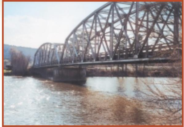
*The two-span, 459-foot Parker truss bridge between Lyme and Thetford, Vermont was completed in 1937.*
