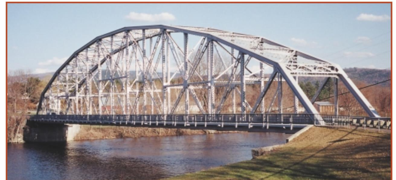
One of the most dramatic bridges constructed after the 1927 flood was the 352-foot Pennsylvania truss span over the Connecticut River from Piermont to Bradford, Vermont, completed in 1929.
